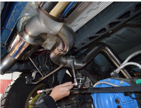
19. If necessary loosen all the clamps and adjust the fitment of the exhaust.
